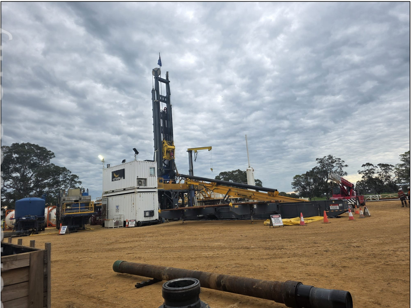
Figure 1: Installation of the surface conductor at Killanoola Oil Field (PRL-13)(October 2025)
