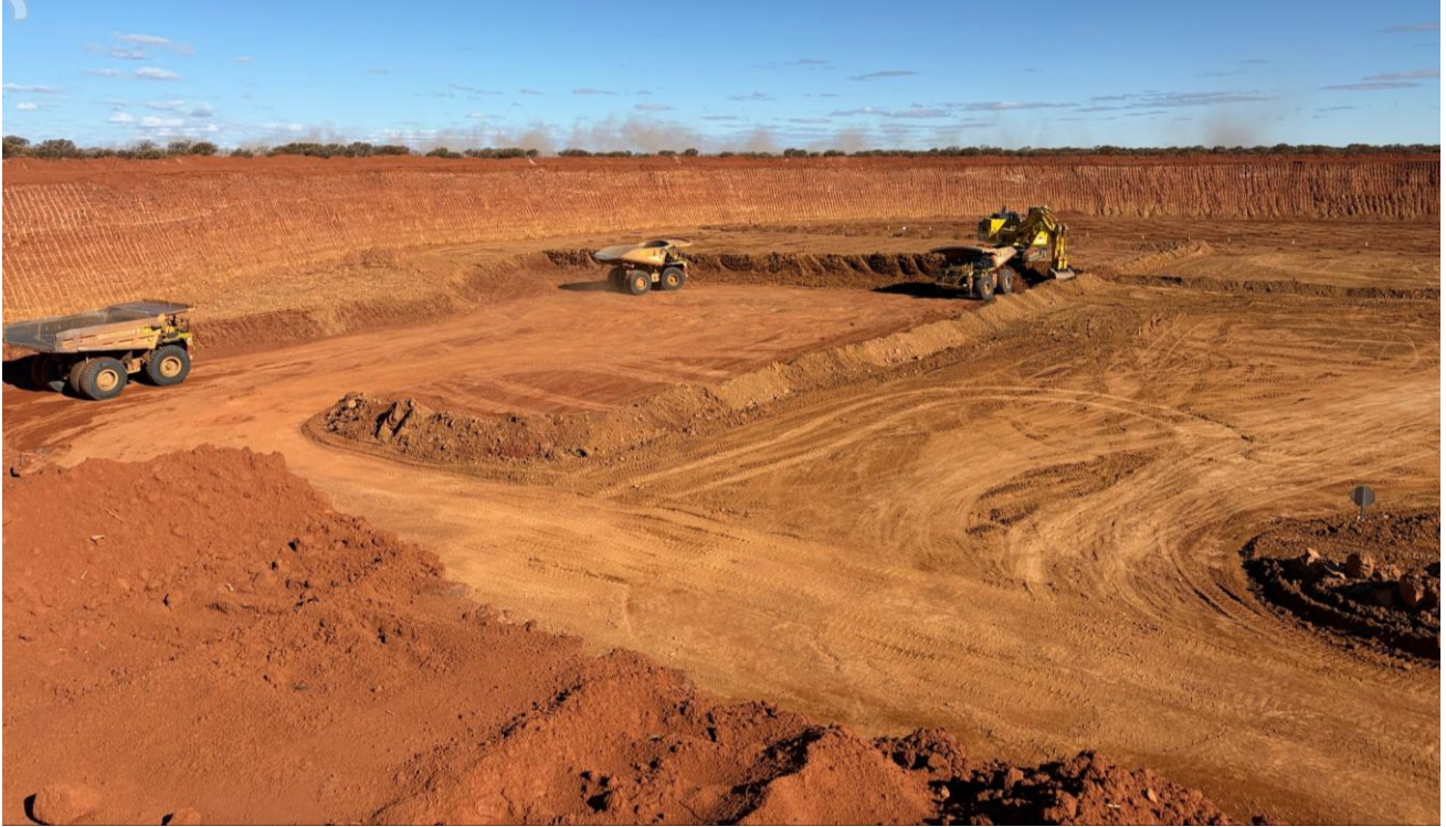
Figure 1: Stripping Stage 1 Turnberry South open pit.
