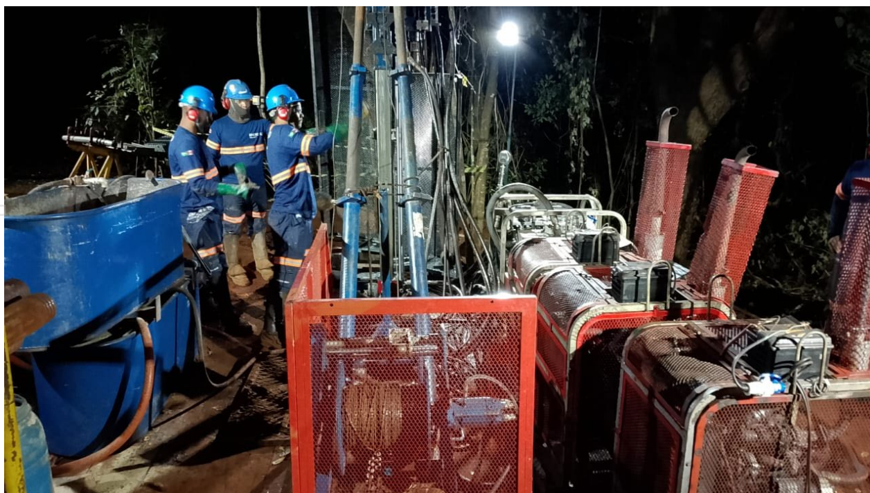
Figure 3 – night shift diamond drilling underway at Araxá.
