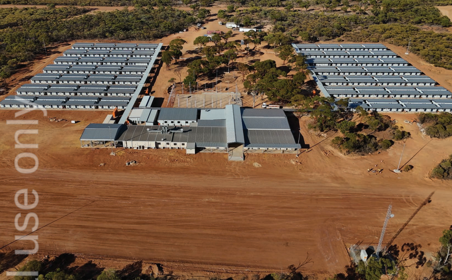
Mt Gibson Gold project – accommodation village installation
