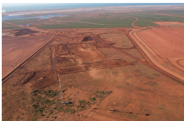
Figure 3: Salt wash plant earthworks commencing
