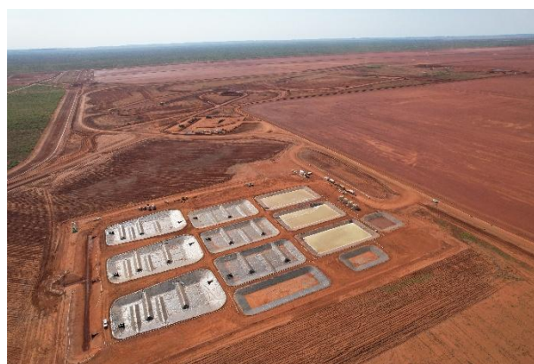
Figure 6: SOP Pilot Ponds being constructed and commissioned
