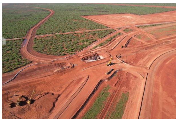
Figure 5: Lift station under construction
