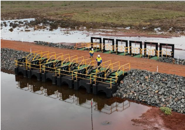
Figure 1: Culvert between pond 7 and pond 8
