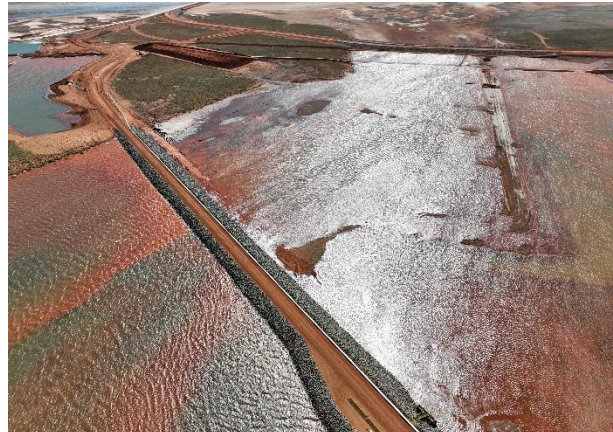
Figure 2: Water inundation at pond 9
