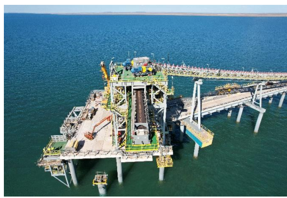
Figure 4: Jetty Head Works nearing completion
