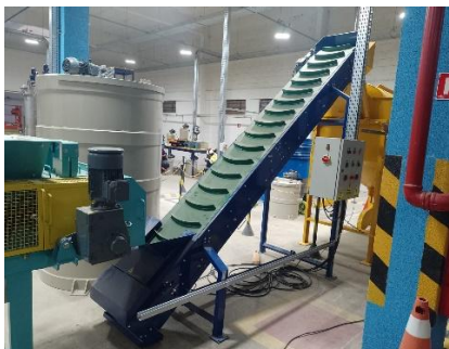
Figure 2: Ore Feed Conveyor leading to trommel
