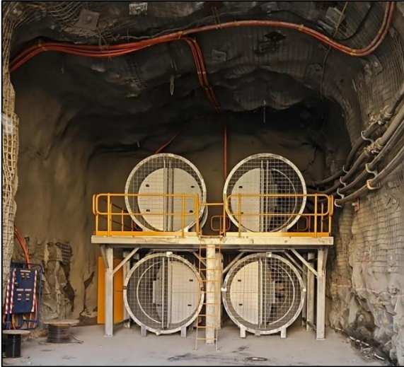
Figure 8 & 9: Never Never underground primary fan installation and first underground electrical sub-station
