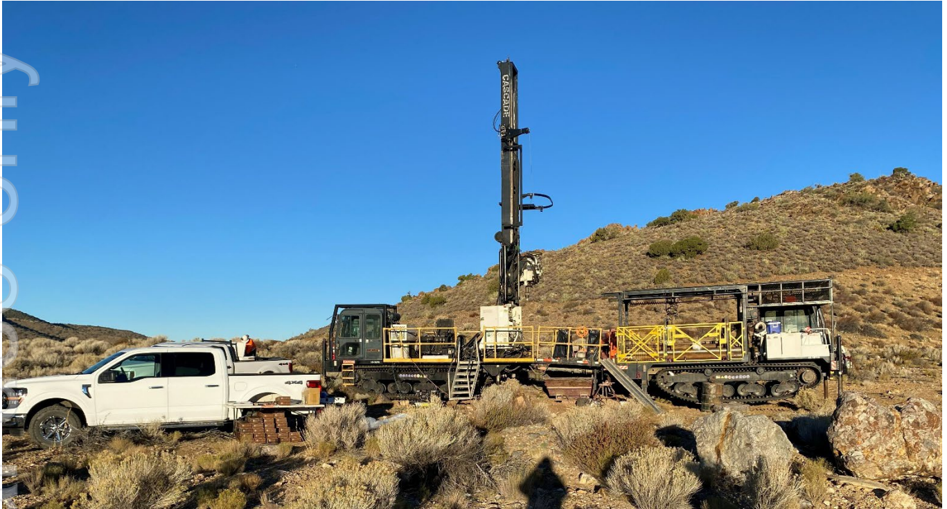
Figure 3: Sonic drill rig on site at the Colosseum TSF
