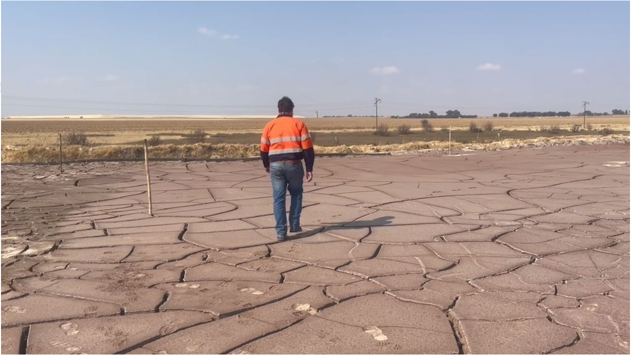
ATA® dewatering enabled rapid consolidation of gold tailings at a South African TSF, achieving trafficable conditions in a matter of days
