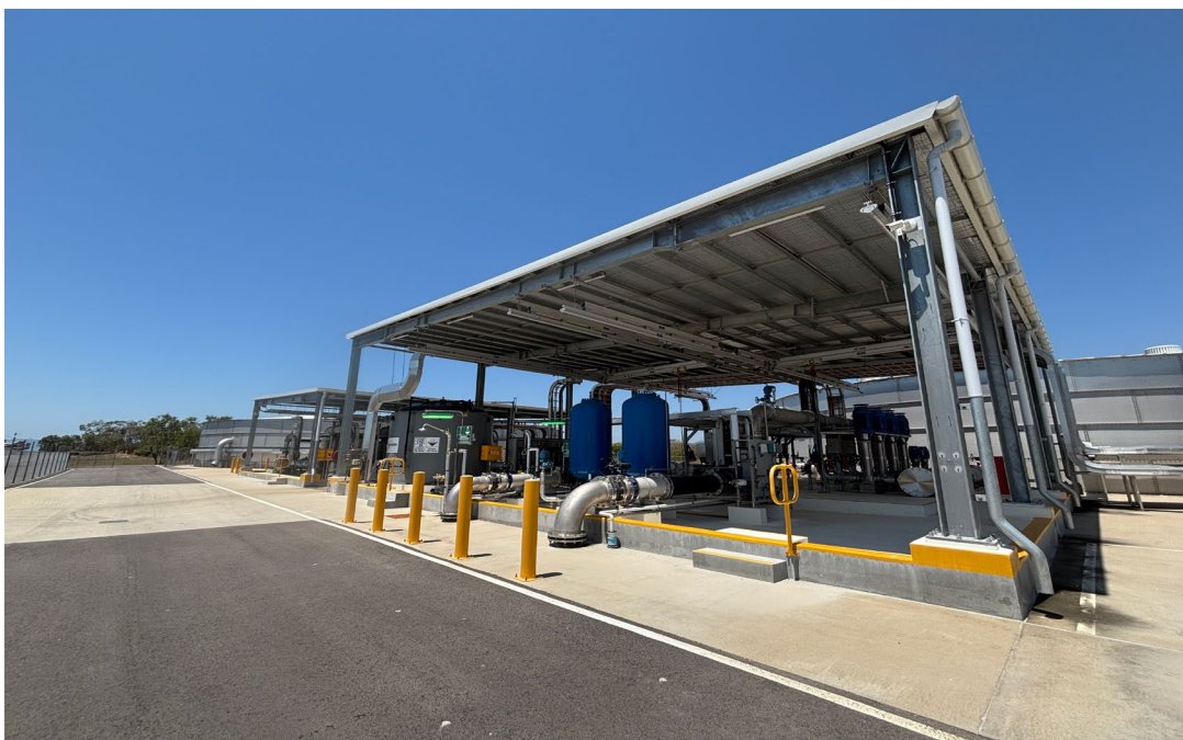
Townsville Water Recycling Facility has achieved practical completion
