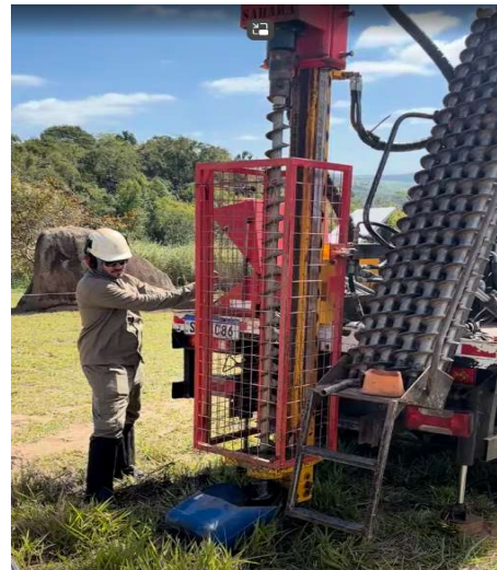
Figure 1: Images illustrating the hydraulic auger drilling process, the systematic collection and arrangement of soil samples for detailed field description.
