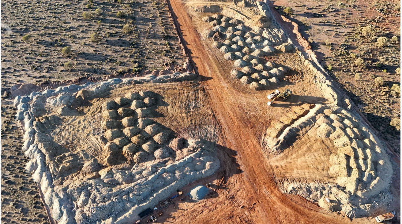
Photo 2: Neta Run-of-Mine/Laydown Stockpile – 25 October 2025
