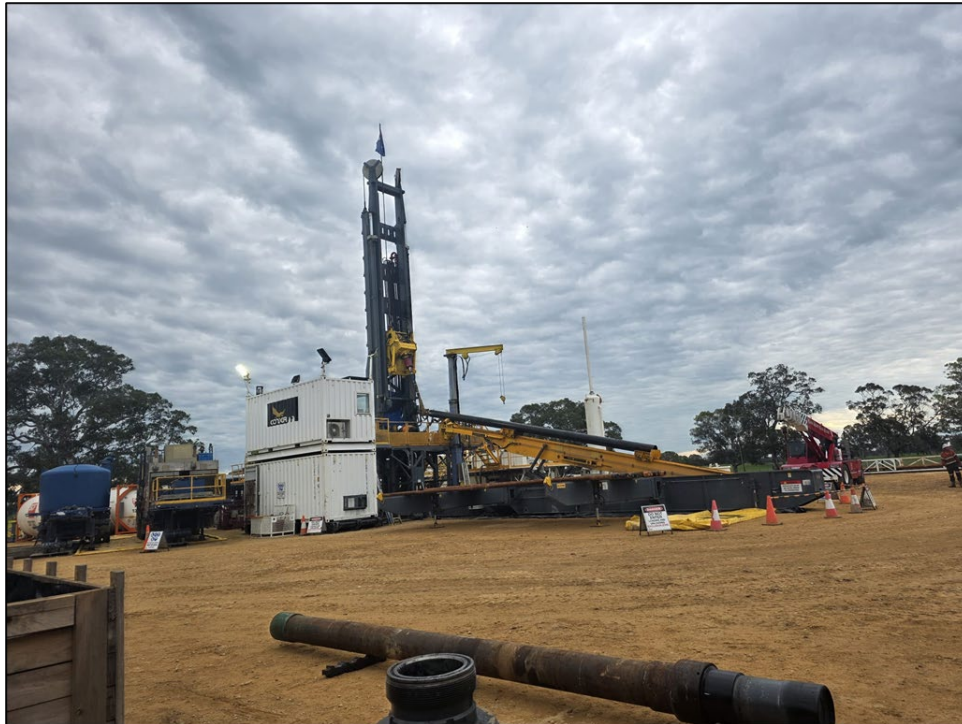
Figure 12: Installation of the surface conductor at Killanoola Oil Field (PRL-13)(October 2025)
