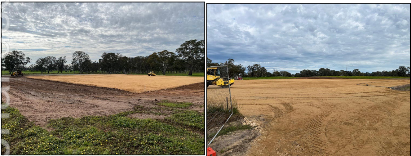
Figures 3 - 4: Well pad completed at Killanoola Oil Field (PRL-13)(September 2025)
