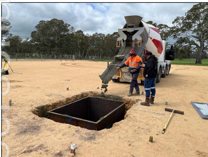
Figure 10 -11: Cellar completed at Killanoola Oil Field (PRL-13)(October 2025)
