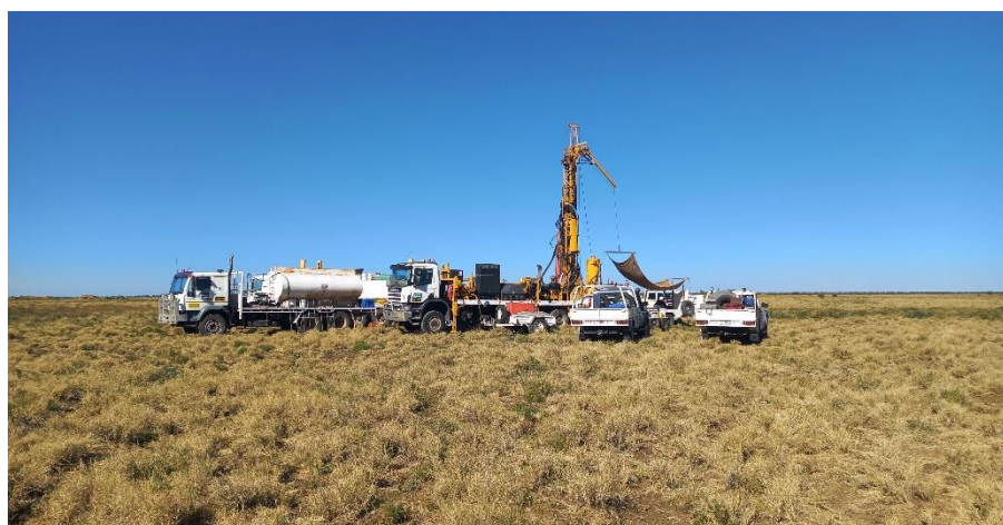
Figure 3: Kilterry2025 Drilling Program works
