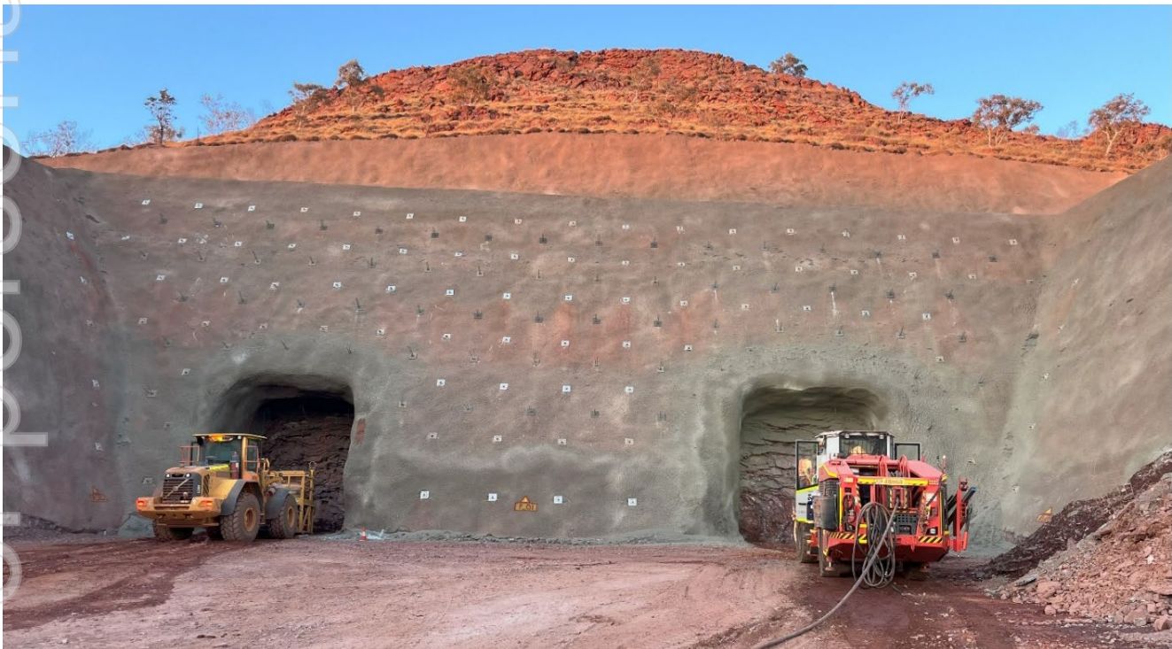
Figure 7: Commencement of Sulphur Springs Exploration Decline and Boxcut
