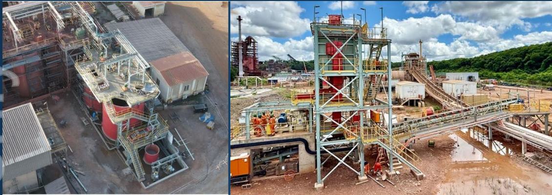
Additional tanks in CCIL circuit and Pebble Crusher circuit
