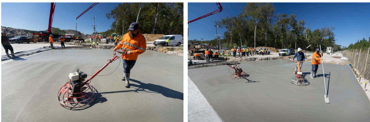
Figure 3: Attendees at the AusPozz™ Commercial-Scale Concrete Demonstration Pour
