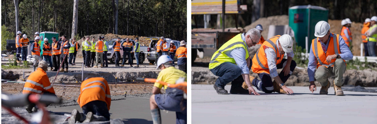
Figure 2: Finishing Work at the AusPozz™ Commercial-Scale Concrete Demonstration Pour
