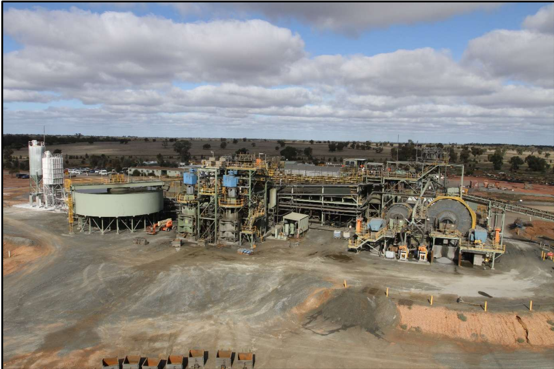
Figure10. The Tritton Ore Processing plant will treat the Constellation supergene, sulphide and high grade oxide mineralisation.
