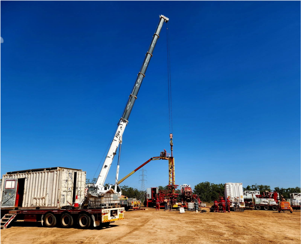
Image: Coil Tubing Unit cleaning out laterals
