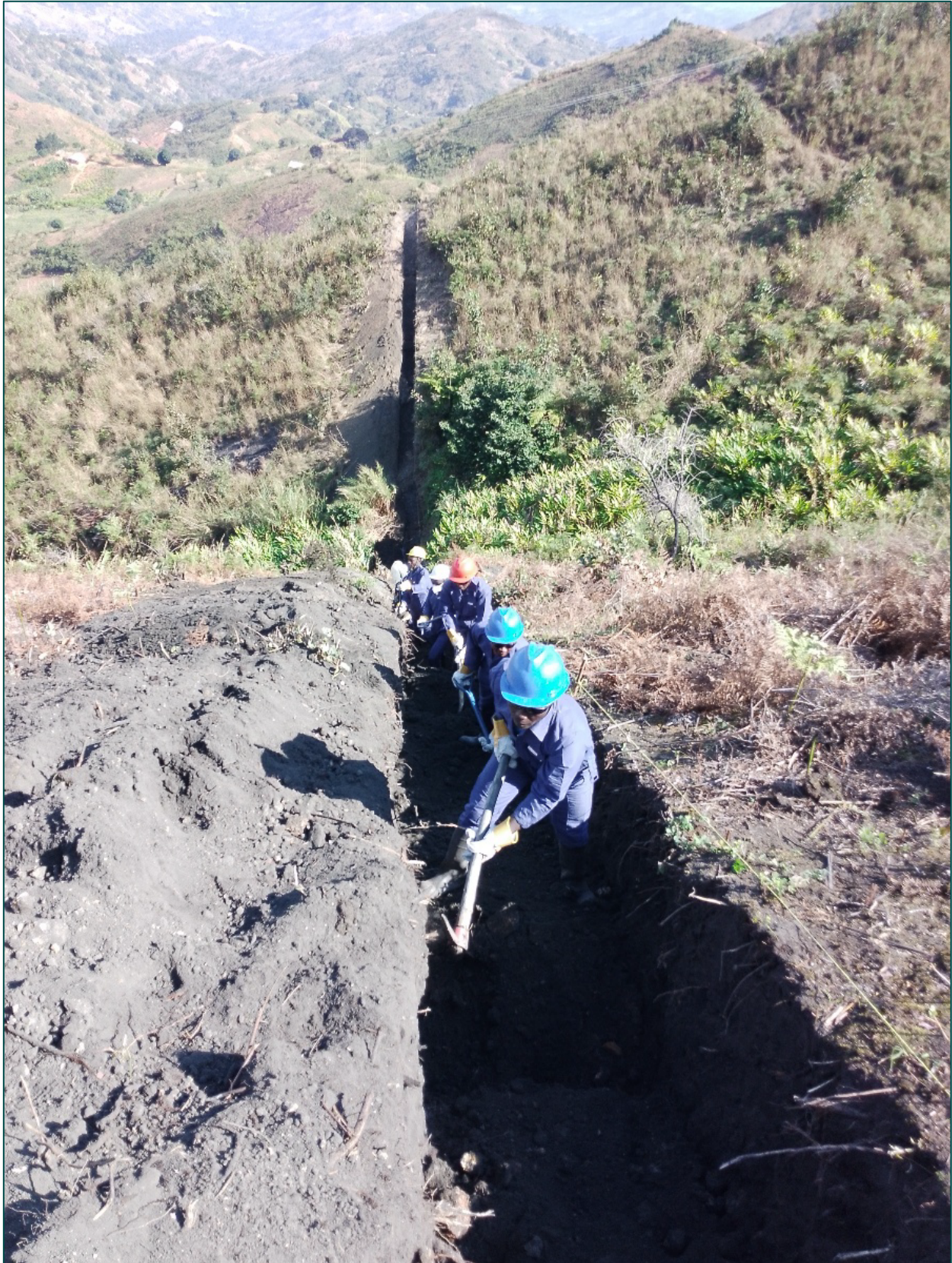
Photo 1: Excavation of trench TRUM23-002
