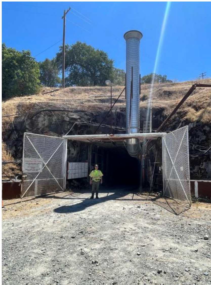
Figure 2: String Bean Alley Decline Unlocked and open for action. The Decline is nearly 900m long, at a decline of 12%, attaining a depth of around 200m below surface. 5
