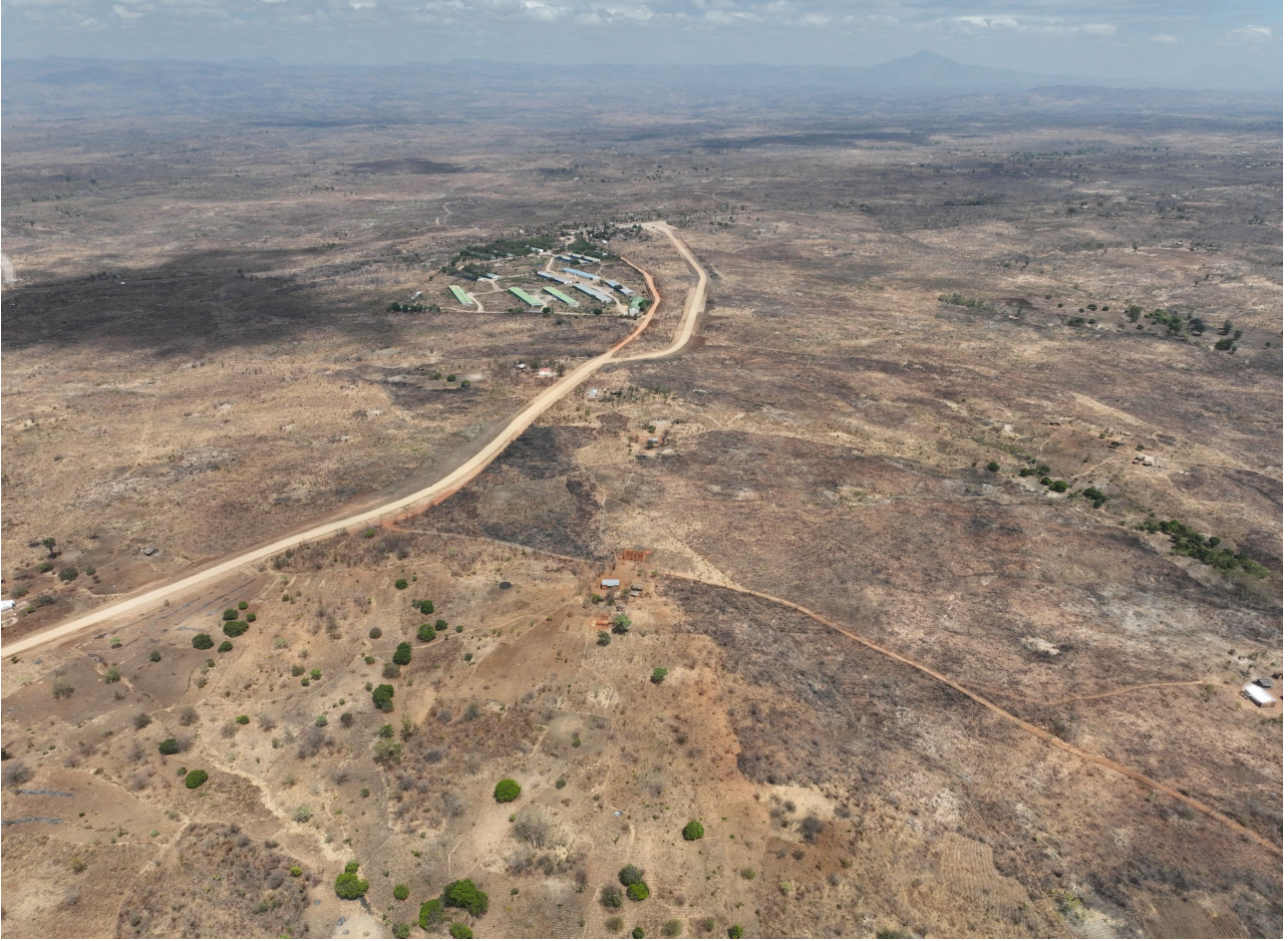
Picture 3. Completed 5.5km access road to site at Kangankunde.
