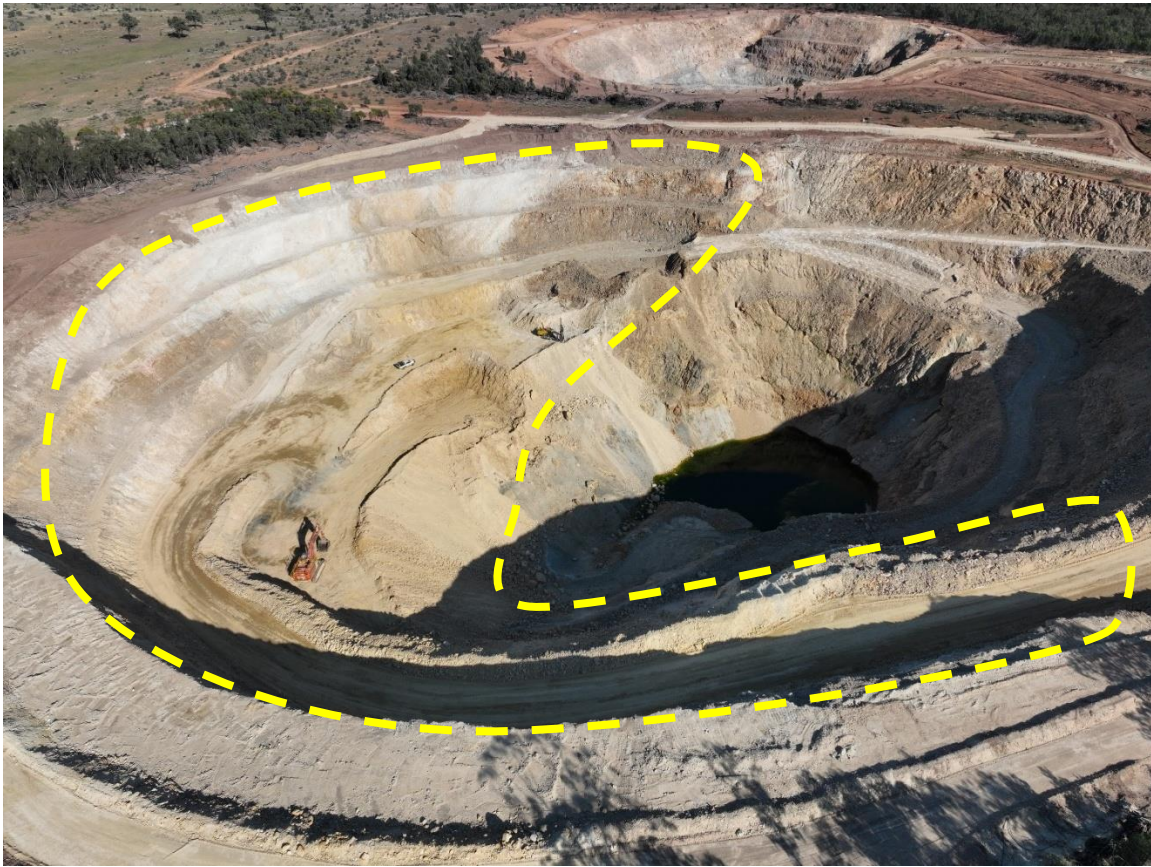
Figure 3: Pearse South open pit progress with Pearse North in the background (ramp and wall cutback outlined).
