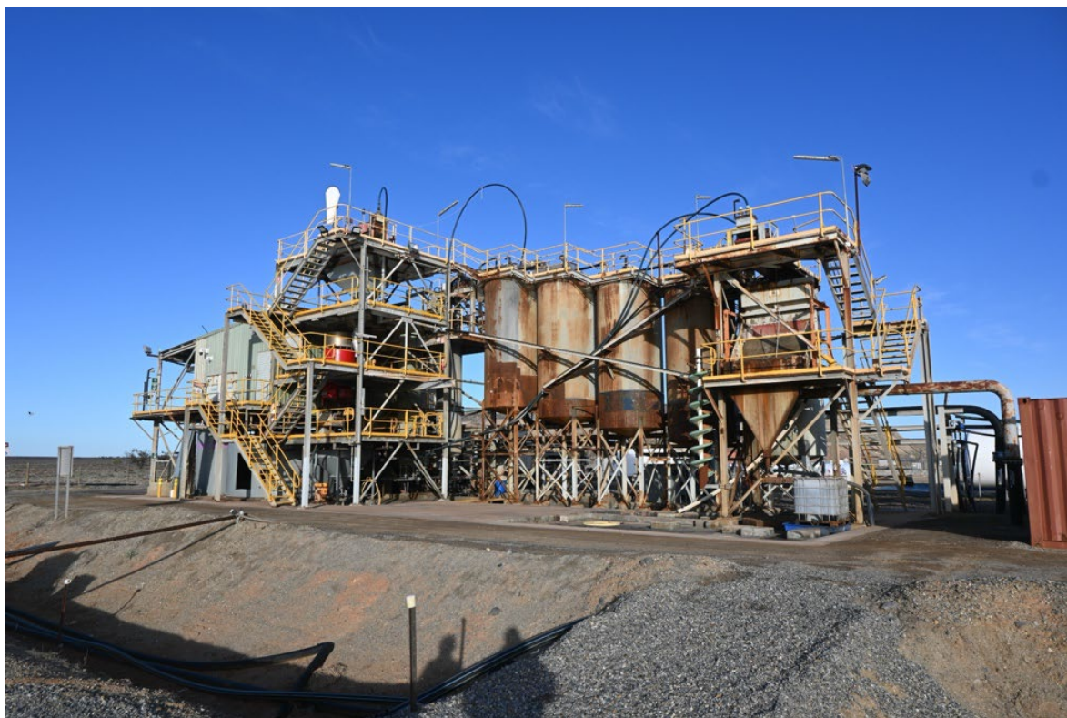
Figure 3: Operating White Dam gold processing plant
