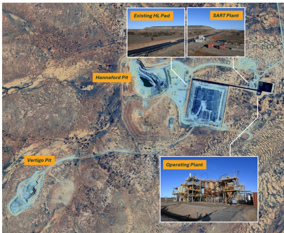
Figure 1: Aerial view of White Dam gold operations site with photos of existing operating infrastructure and heap leach pad
