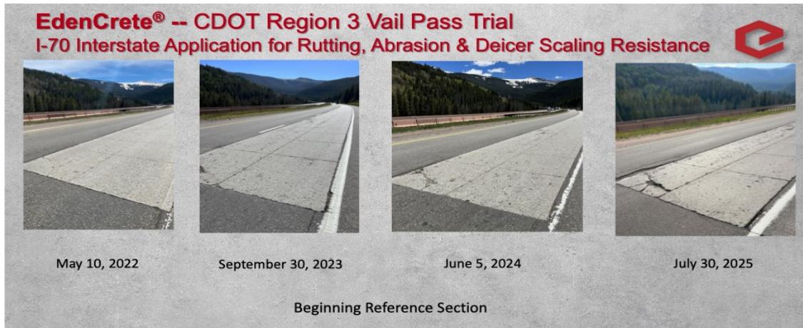
Figure 7. Standard Portland Concrete Reference – Beginning Section
