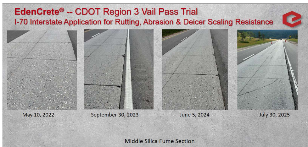
Figure 11. Silica Fume concrete – Middle Section
