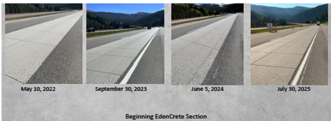
Figure 6. EdenCrete enriched concrete – Beginning Section
