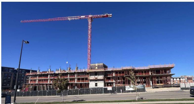
Figure 1. The Bellview Station Block F project- progress to date.
