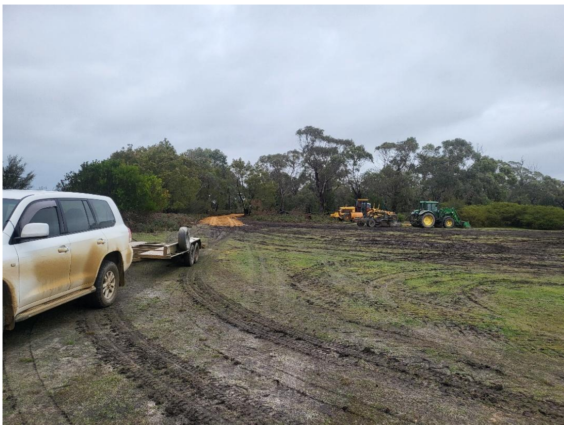
Figure 1: Early site works at Wombat-5
