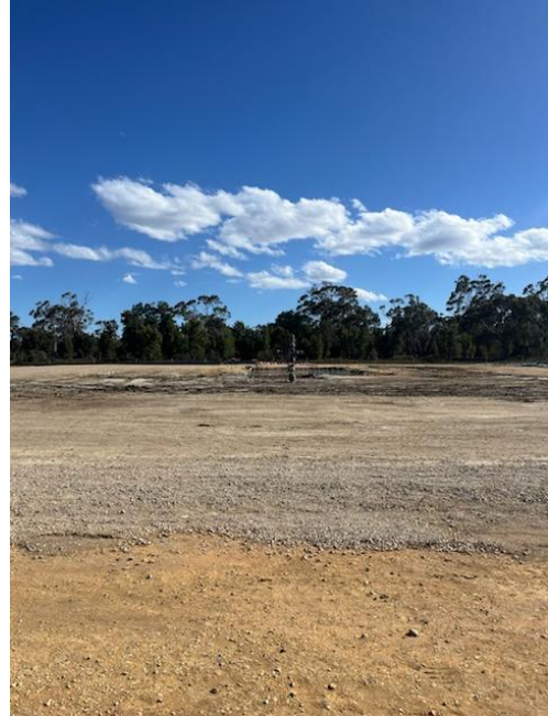
Figure 3: Cleared Wombat-5 site post-demobilisation
