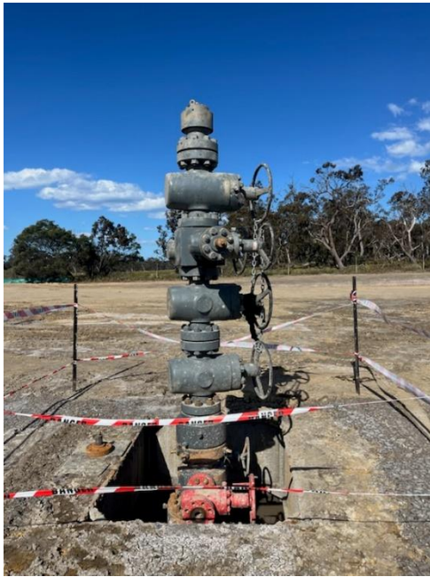
Figure 2: Wombat-5 wellhead installation
