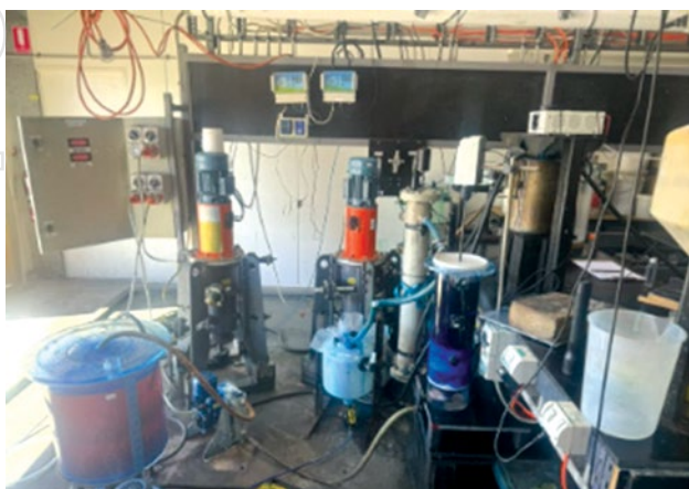
Figure 4 – BHTC's cobalt solvent extraction circuit
