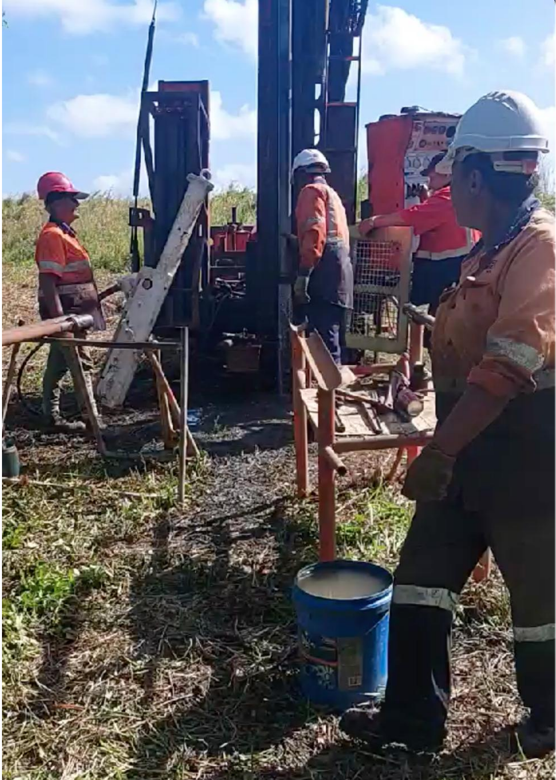
Plate 1 – Geotech drilling program at Kulukulu South sand processing plant site
