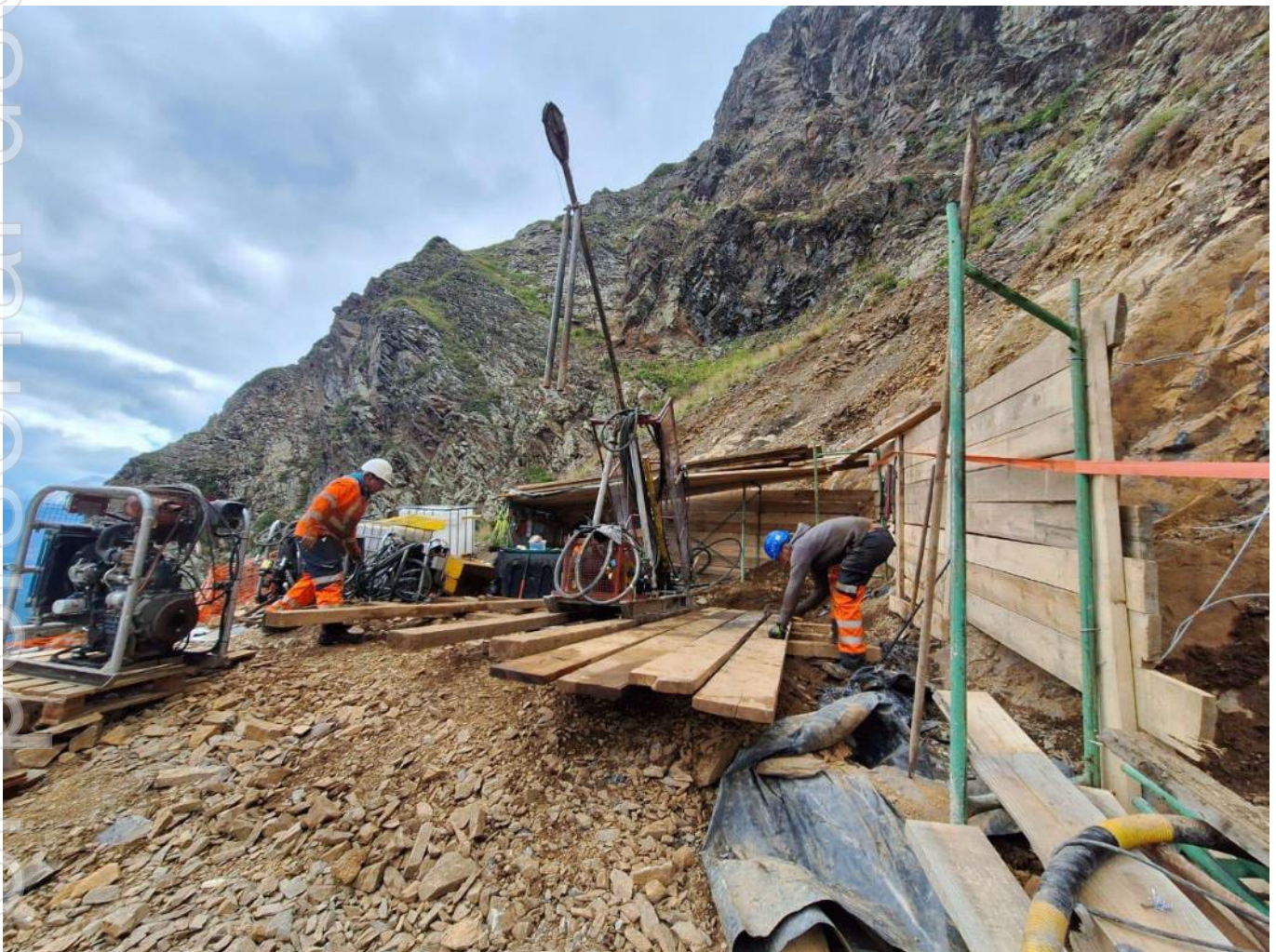
Photograph 1 - Man portable diamond drill rig being prepared for drilling on platform 2
