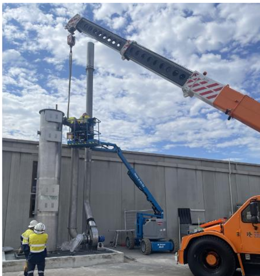
Figure 4. Installation of scrubber at PSG demonstration facility
