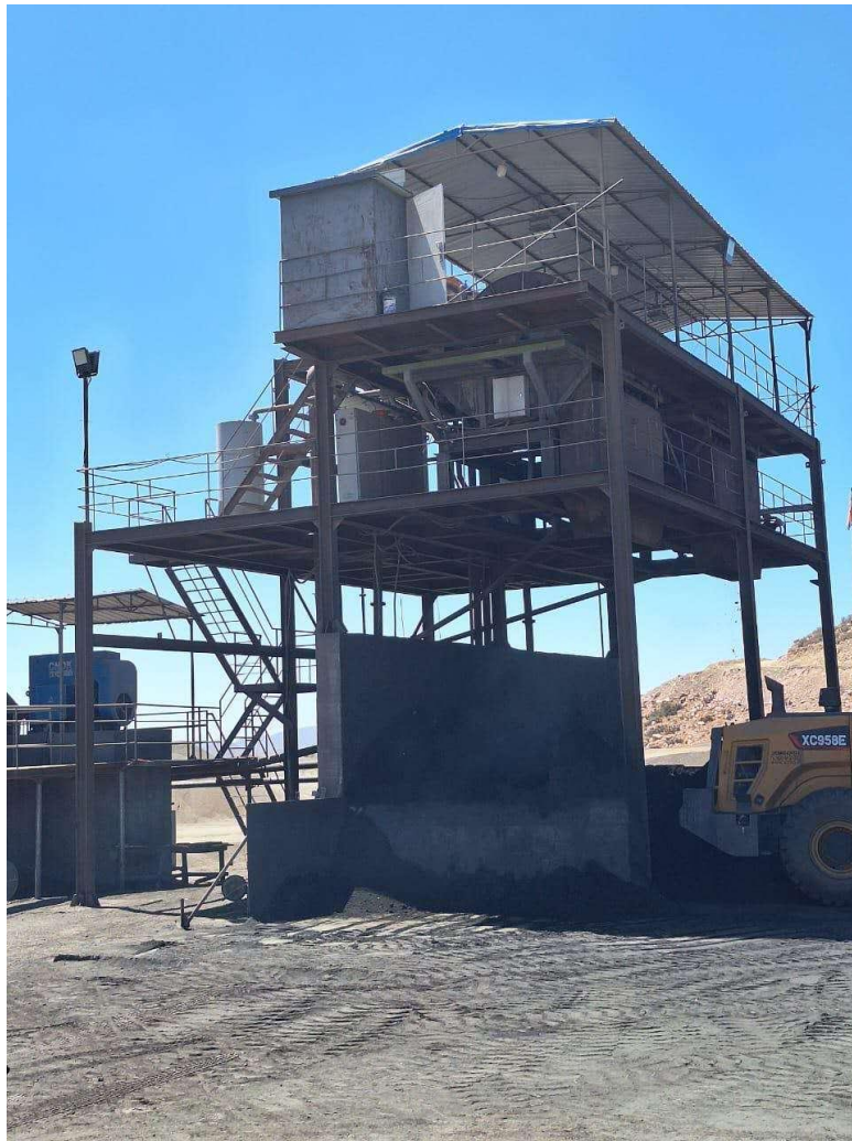
Figure 2: Third stage of crushing
