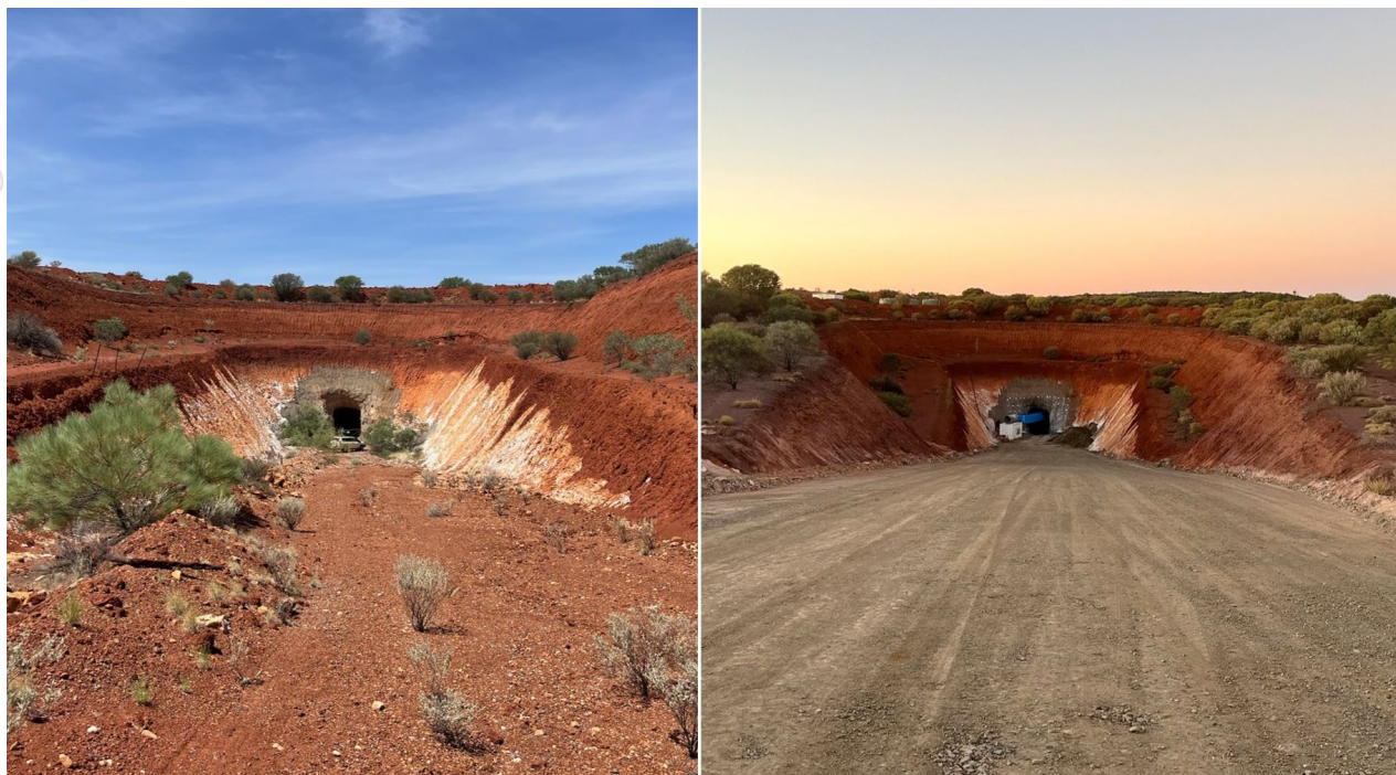
Figure 8: Refurbishment of K2 boxcut and portal
