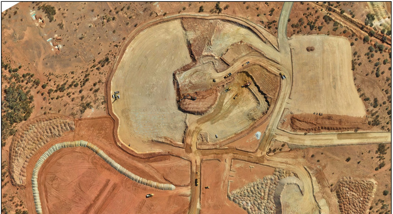
Figure 7: Trident open pit progress during September
