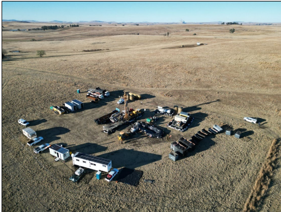
Figure 1: Drilling rig on site for drilling commencement well 271-KA03PT06
