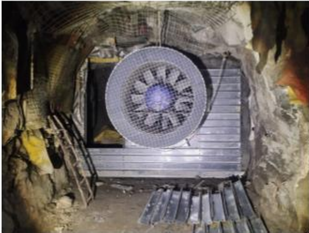
Image 8: Installation of 110kW ventilation fan
