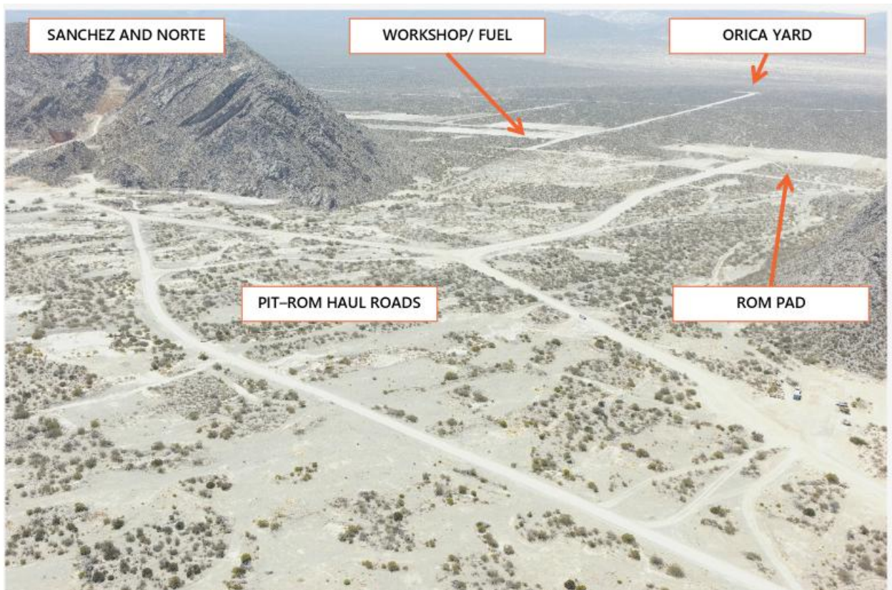
Figure 2 - Expanded View Cerro Norte showing Infrastructure (taken 2 weeks ago)
