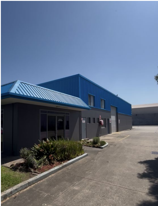
Image 2. Prefabrication Facility in Penrith, NSW
