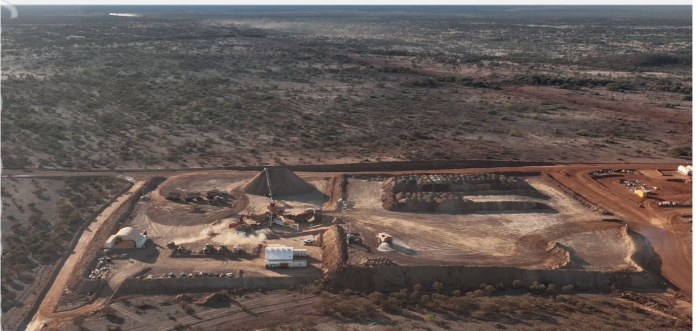
Figure 2: Crown Prince ROM and Crusher Pad
