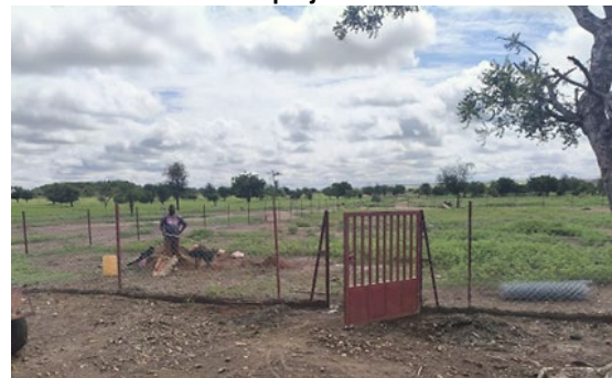
Fence construction at market garden extension project
