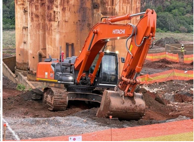
Figure 9: Excavation work for Gold Room
