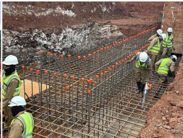
Figure 5: Steel reinforcing installation and preparation for concrete placement
