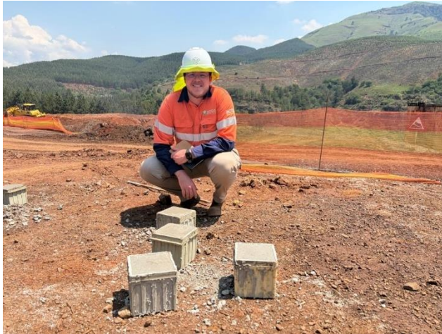
Figure 2: Engineering inspection of concrete test cubes
