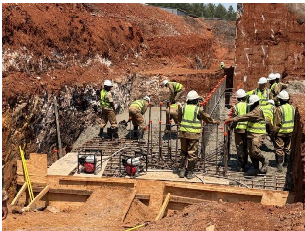
Figure 6: Placement of concrete foundation for terrace wall
