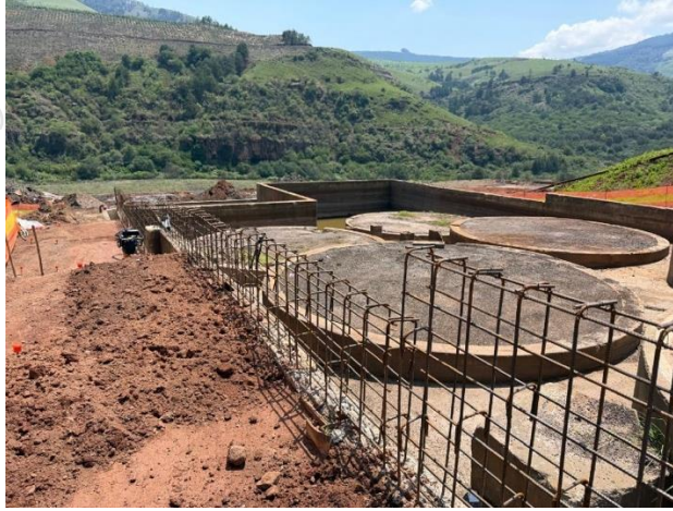
Figure 8: Steel reinforcing installation at CIL section
