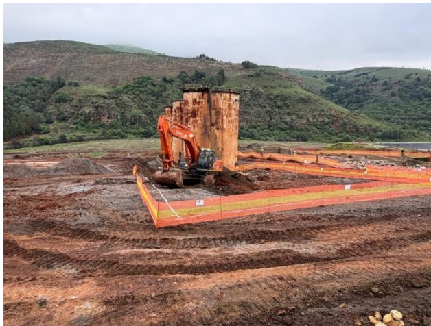
Figure 4: Earthworks for the gold room foundation works
