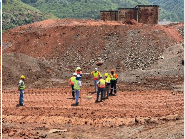
Figure 3: Project team taking soil compaction tests
