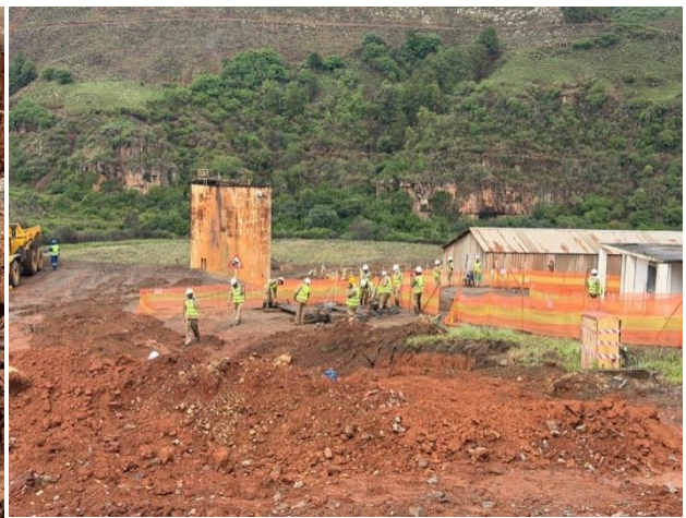
Figure 7: Transporting of steel reinforcing for CIL bund wall extension
