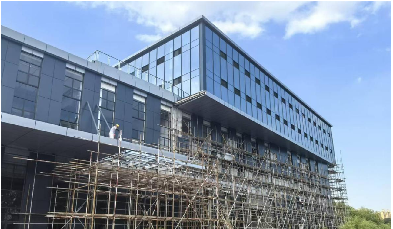
Photo: Vmoto's new manufacturing facilities in Nanjing, China under construction.
