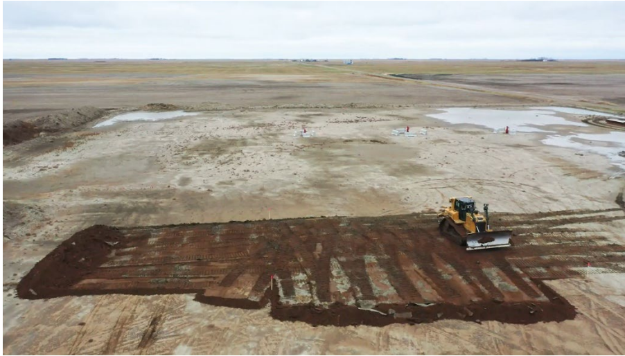
Figure 1: Foundation works on Pad #1
