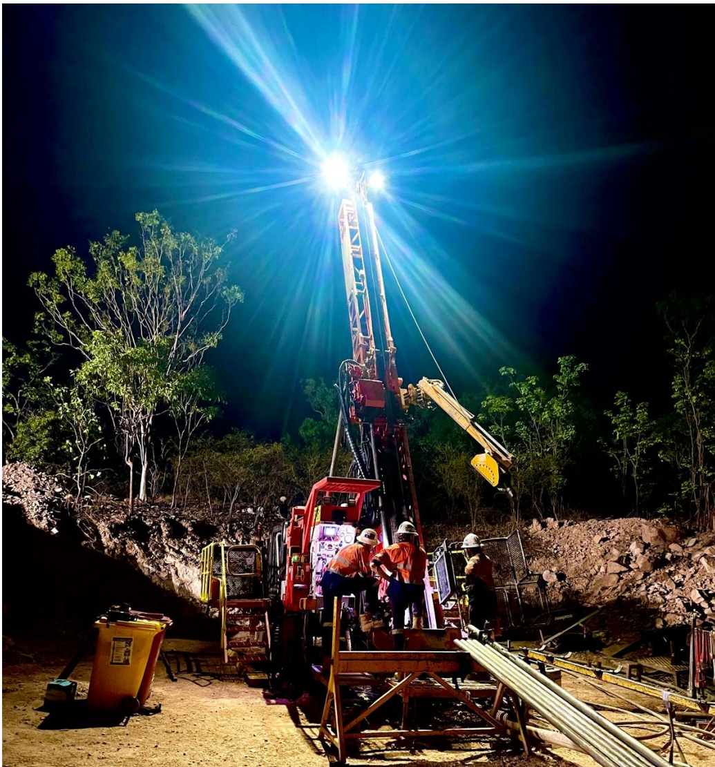
Figure 1: DDH 1 Diamond Rig onsite at Spring Hill
