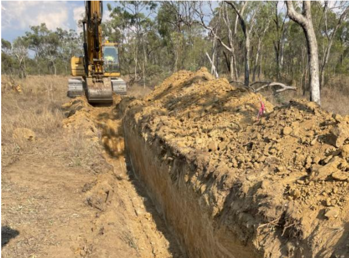
Figure 1 – Trenching underway at Oasis, structural measurements and radiometric data is recorded after each trench is dug, trenches are then backfilled and rehabilitated.
