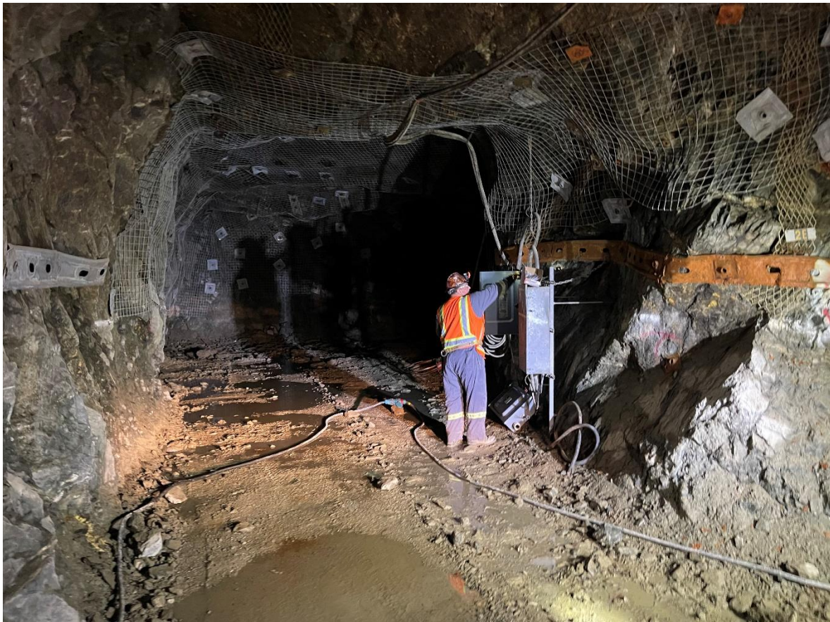
Figure 1: Recently drained XC2 being prepared for temporary storage of MPC to transfer power down Stringbean Alley Decline.
