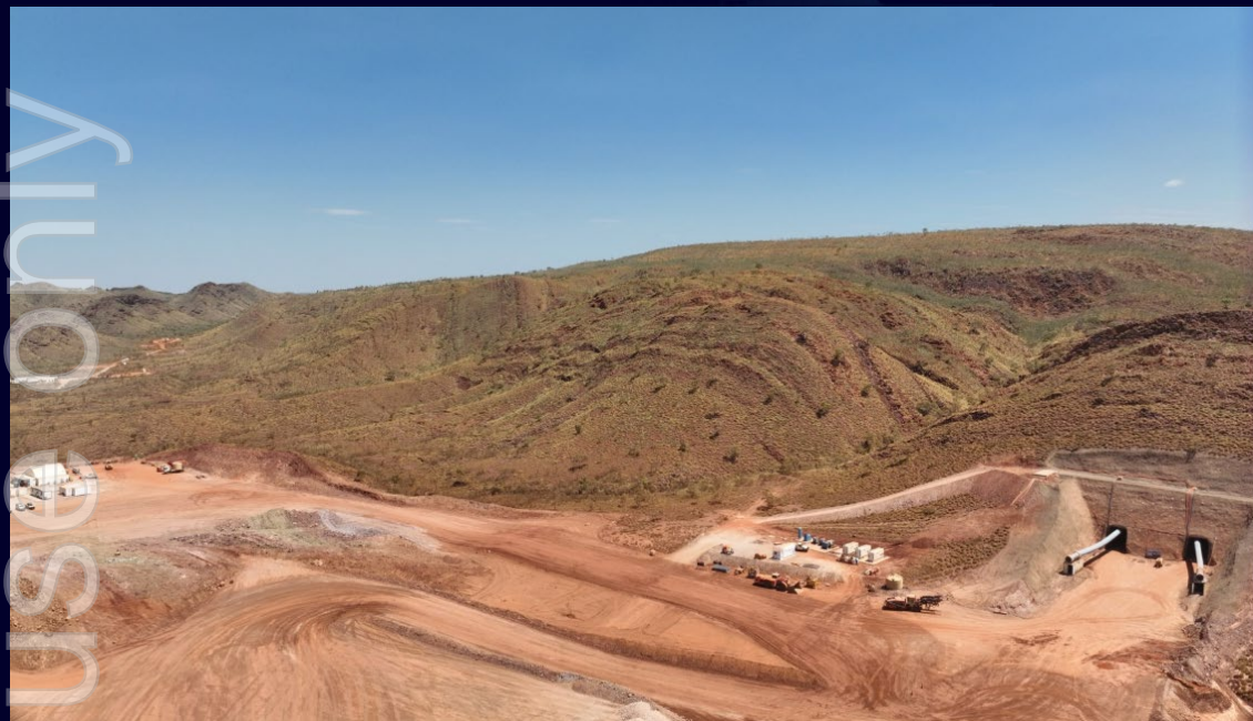
Box cut complete, twin declines started, UG service workshop set up, site infrastructure locations cleared
