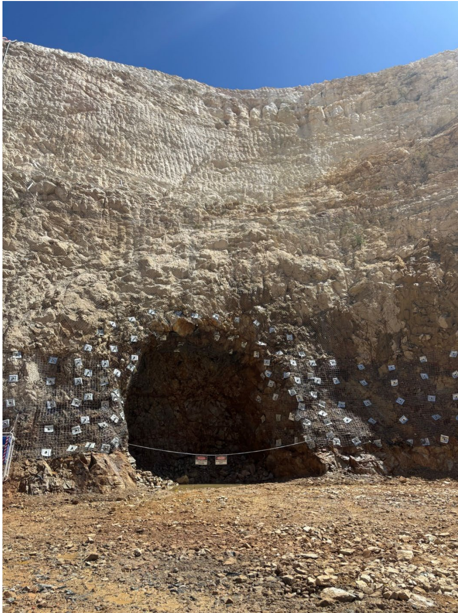
Figure 3 – First cut supported
