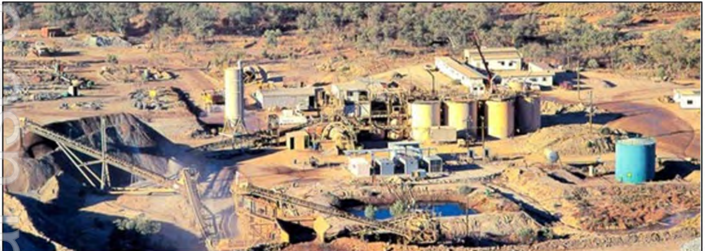
Figure 2.3 - Butchers Creek Gold Processing Plant 1996
