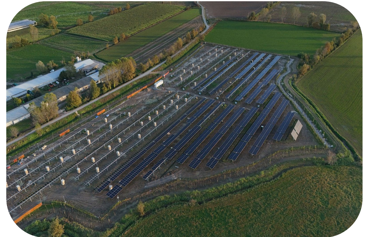
Galileo's solar project under construction in the Lombardy region, Italy.
