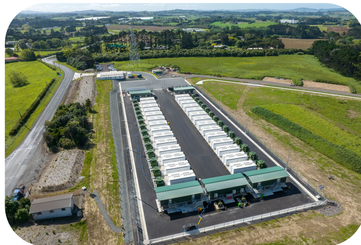
Contact's 100MW battery facility located at Glenbrook in South Auckland
