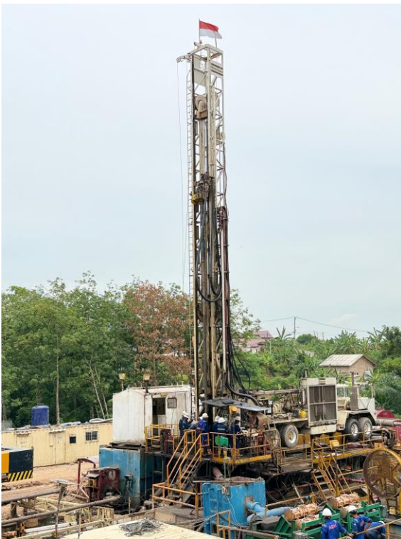
Drilling Activity TE B01-003
