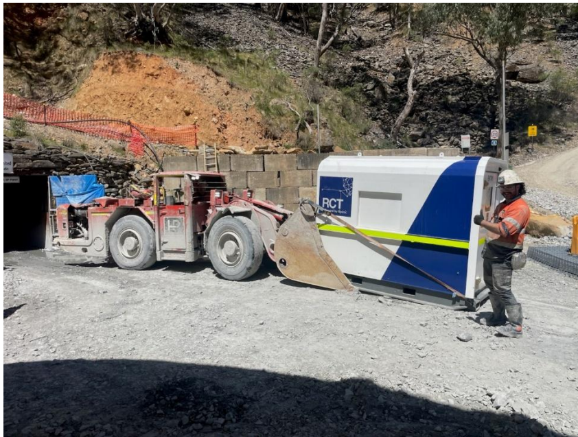
Figure 1 – Tele-hut being taken underground
