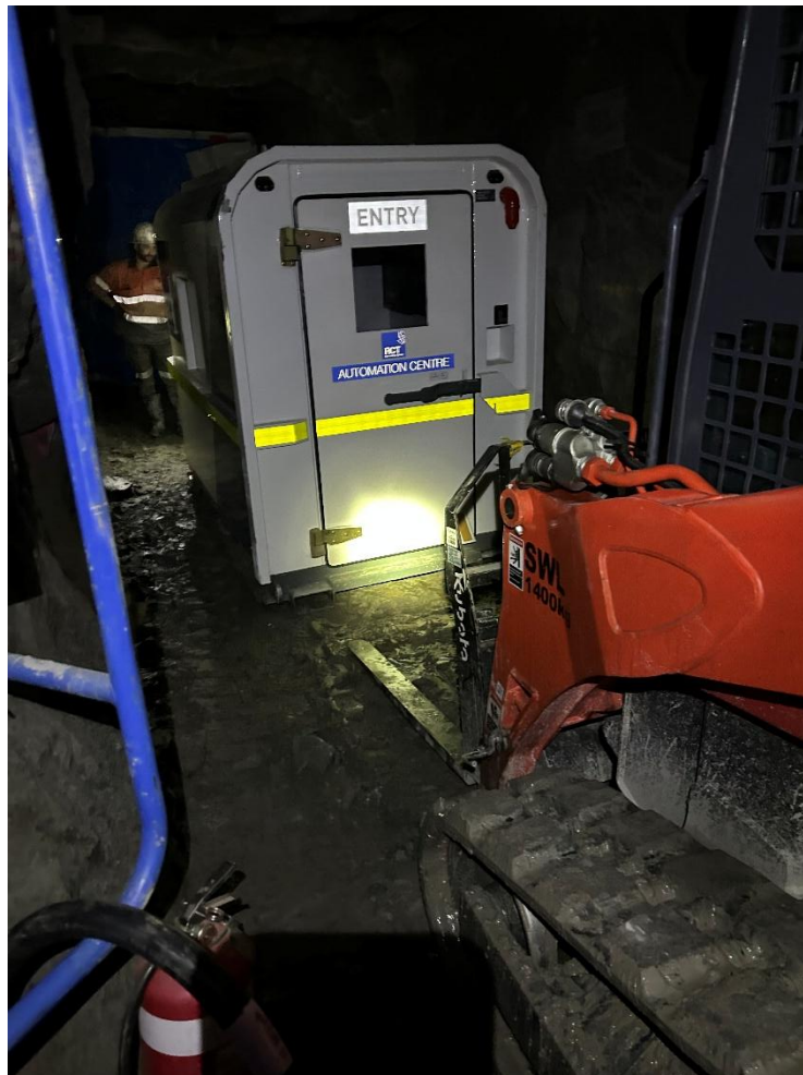
Figure 2 – Tele-hut installed underground
