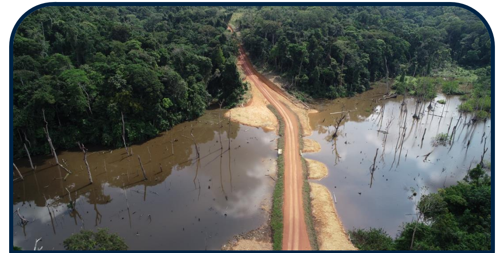
Resurfaced Tsengué Base Camp access road.
